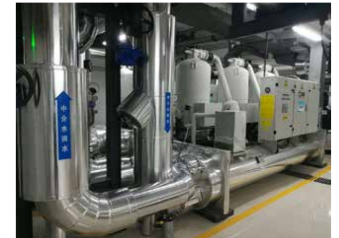
Figure 25. Heat pump in Uni Town, photo credit: City of Qingdao.
